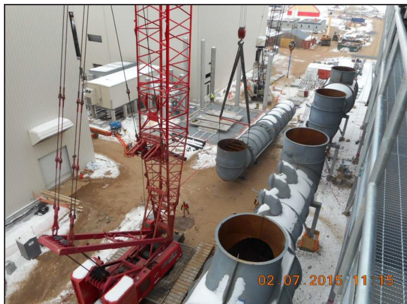
Figure 12 Actual Structural Loading During Installation
