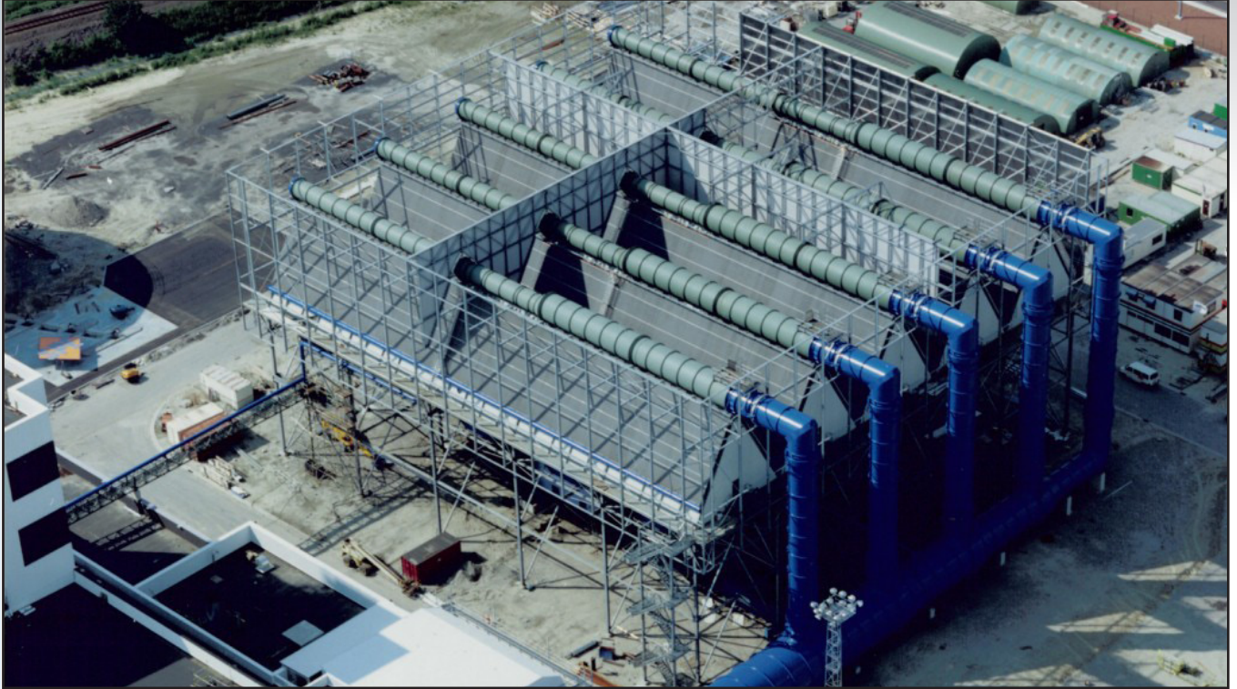
Figure 1 Typical Air-Cooled Condenser
